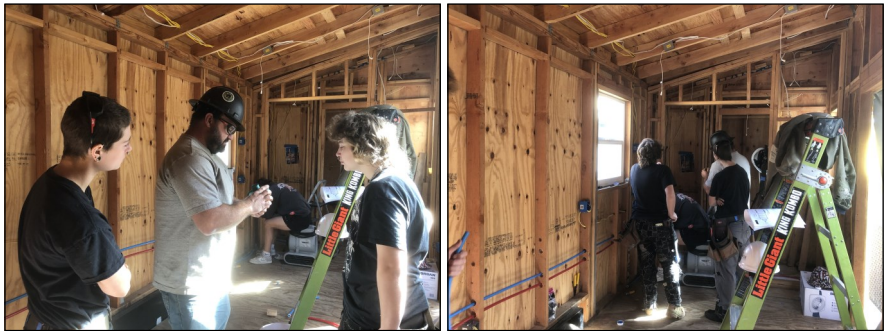
The A Team at work installing rough plumbing.
