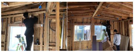
On rainy days a few students worked inside our cottage checking items off of their 'punch list'. In late January, two student builders were installing additional blocking at the intersection of the walls and ceilings around the inside perimeter of the house to support the 'hanging' of dry wall.
