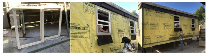
The first course of siding takes awhile to position correctly. But, after the first course is in place, the subsequent courses go up pretty quickly. The team uses clamp-on siding gauges to ensure that each course of siding overlaps the previous course by a consistent amount.
