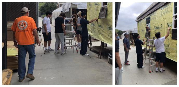
Using the James Hardie fiber cement trim boards donated by <u>Weyerhaeuser</u>, our students fabricated corner pieces for each corner of the house. The siding on each side of the house will 'die into' or 'butt up to" the corner pieces.
