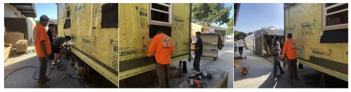
While one team of students was installing siding, another team was in the workshop building wood window frames. They used a pocket-hole machine in the workshop to drill holes for screws in the back of the 4 frame pieces. After assembling the frames and positioning them around the windows, they took measurements to make sure that they hit studs when they attached them to the house with screws.
