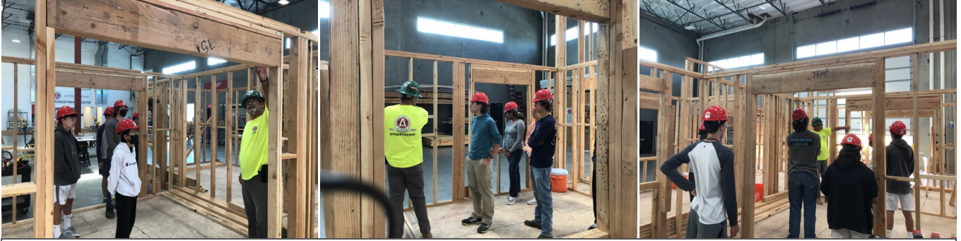
Alan Jurgensen explains the design of wood frame structures before the students start framing a wall.
