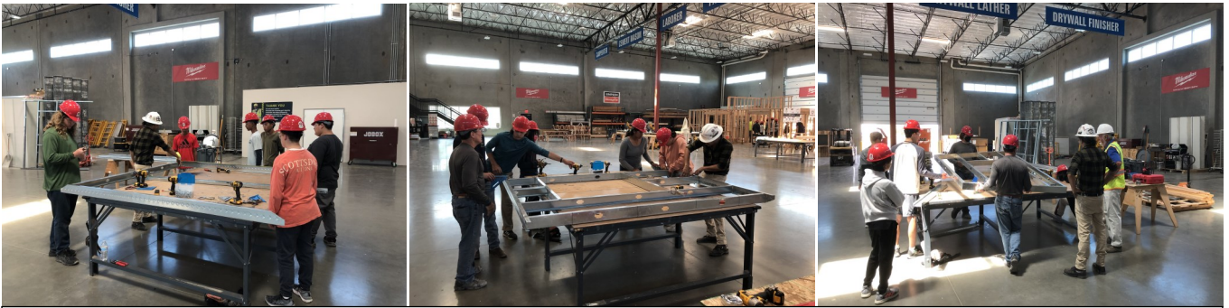
Chris Griego demonstrates how steel studs are used to frame a wall.
