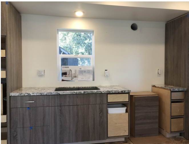
Our beautiful granite countertop installed.
