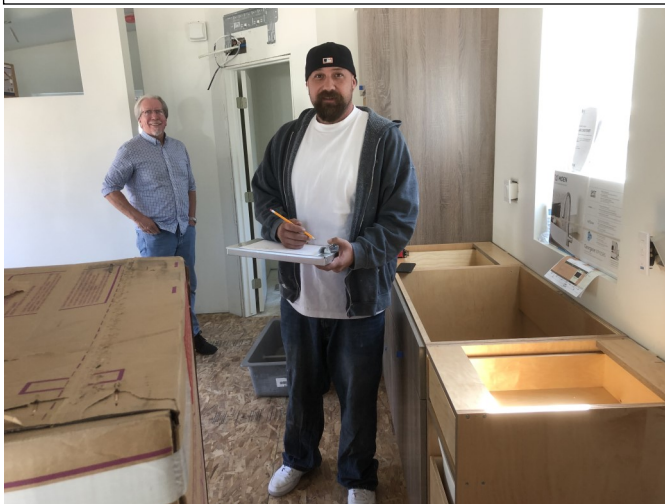
Jesse Esparza of So Cal Counterworks came to the site on November 9 to take measurements for the countertop that So Cal would fabricate from the granite slab donated by Arizona Tile . Jesse's measurements were translated into a construction drawing by So Cal's drafting department.
