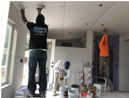
Mesh tape on ceiling butt joints.
