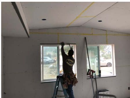
David measures, cuts & staples corner bead around windows. Sergio applies mesh tape on corners.
