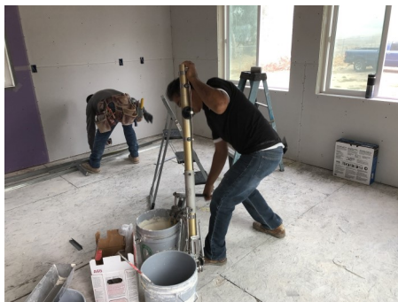
Raul loads his Automatic Taper and lays a bead of joint compound and paper tape.
