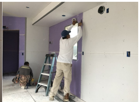
David measures, cuts & staples corner bead around windows. Sergio applies mesh tape on corners.
