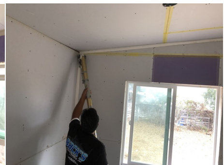
Raul loads his Automatic Taper and lays a bead of joint compound and paper tape.
