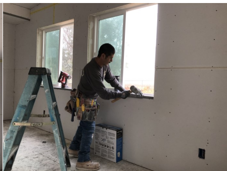
David measures, cuts & staples corner bead around windows. Sergio applies mesh tape on corners.
