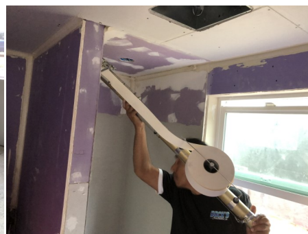
Raul loads his Automatic Taper and lays a bead of joint compound and paper tape.
