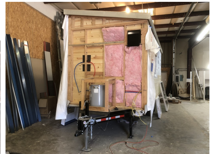
Photos, clockwise from upper left: Southwest High's trailer foundation; CAD drawing of 2" x 4" wood framing for tiny house; rake wall, insulation and water heater; wood frame of similar house under construction.
